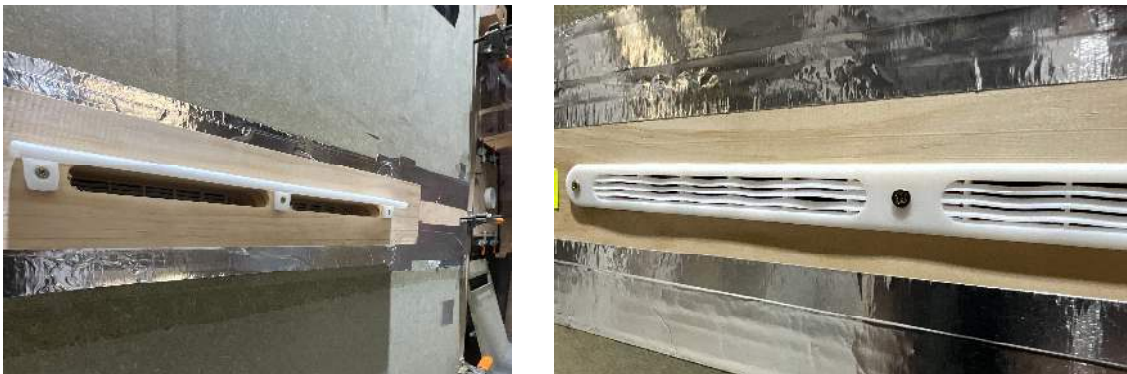
Figure 2 Vent installed onto block and in board of plenum.
