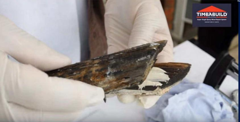
ERC10 is being used as an adhesive to a fascia end section
