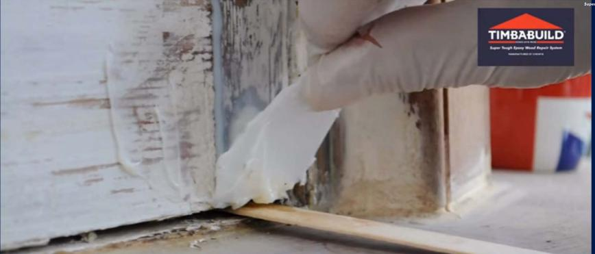
EHB60 is a 'structural marine grade' anti-slump, flexible epoxy resin
