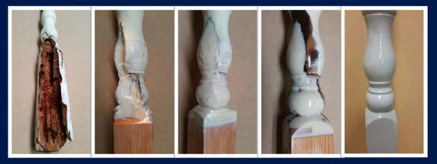
EHB60 is a 'structural' anti-slump resin which can be builtup and shaped to match existing timber structures
