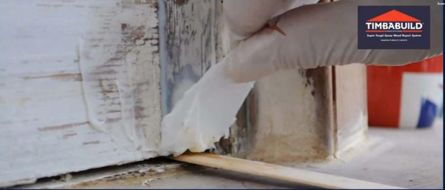
EHB60 is ideal for filling large cracks and holes to existing timber structures.
