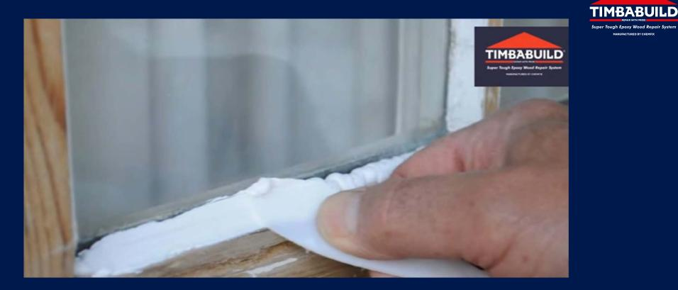
Once extruded onto surface, smooth over using a small scrapper or damp finger to fully seal glazing unit.
