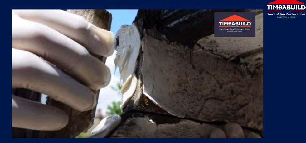
The ERC10 acting exactly like a glue; broken timbers are able to be pieced together again
