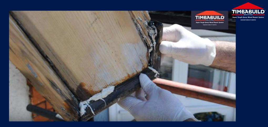
As ERC10 is a rapid setting epoxy, ensure timbers are placed in the exact position to set
