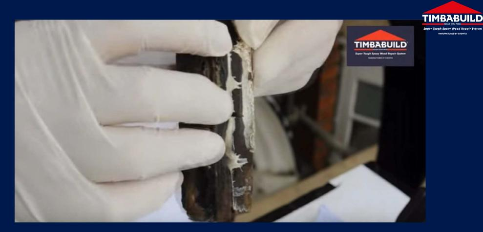
The fast gelling nature of ERC10 makes it ideal for this kind of adhesive repair or for emergency call-out repairs
